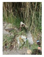
Figure 7: leaking water pipe
